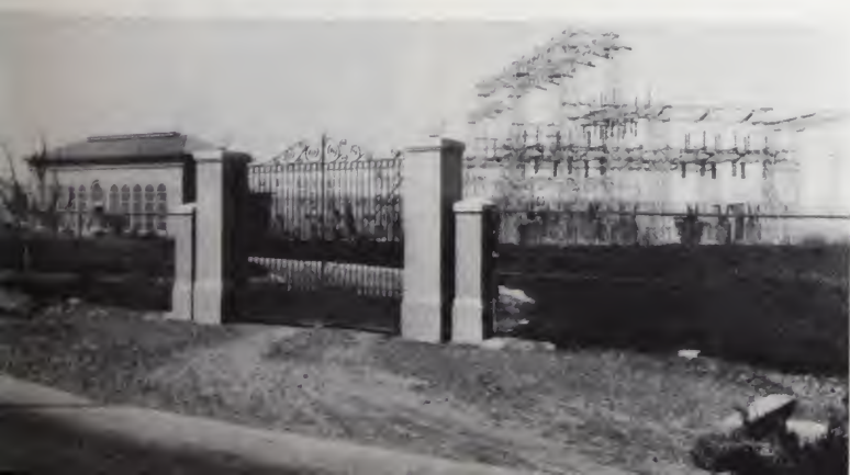
Here is still another example of a Cyclone Safeguard Fence enclosing an electric power station. Note the high steel picket gate set between stone posts. See how well the trim Chain-Link fabric and the graceful steel picket gate set each other off, yet combine in a most attractive and effective enclosure.
